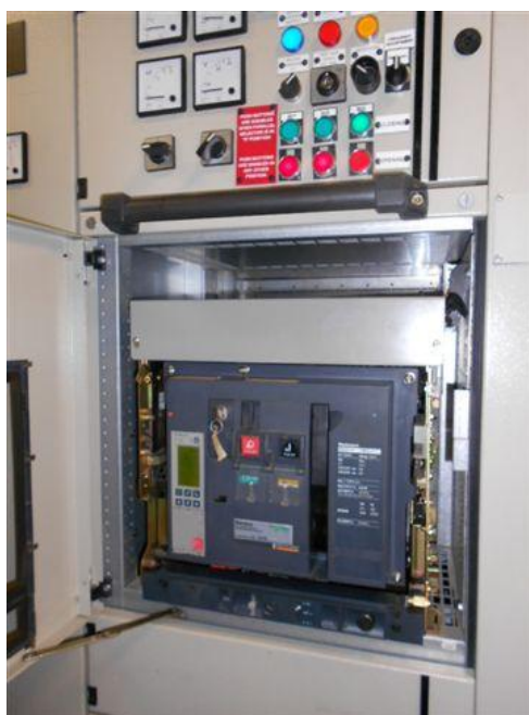
Switch nr. 901 (picture taken from Costa Favolosa)
